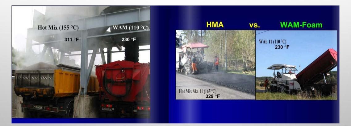
In the HMA the maximum amount of RAP it is strongly related at working temperature: in a lot of cases temperatures are too high with risks for the quality of the added bitumen (early aging) and big increase of costs and emissions
